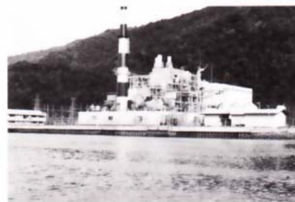
A view of the Khanom Thermal Power Plant.
