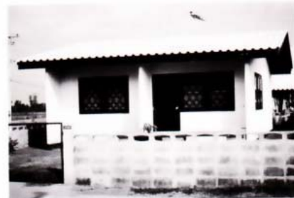
Typical low-cost dwelling unit at Buakhoaw Estate in Minburi District, Bangkok.
