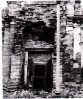
Deterioration of Wat Prang Khaek in Lopburi province.
