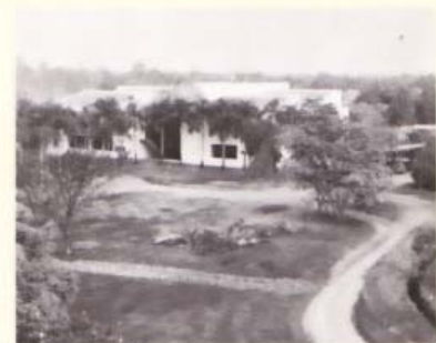
Clearing of site for the Outreach Building.
