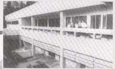
Left: The middle section of the Administration Building prior to the addition of a second floor (above). Below: The AIT Center annex and its beautiful gardens.
