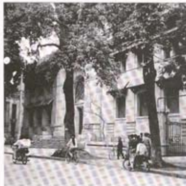
AITCV's temporary office in Hanoi.
