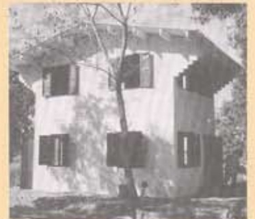
Above: Construction of the Aquaculture building using prefabricated building components developed and produced by the Habitech Center. Some of the prefabricated components are similar to those used in the Habitech demonstration house (right).
