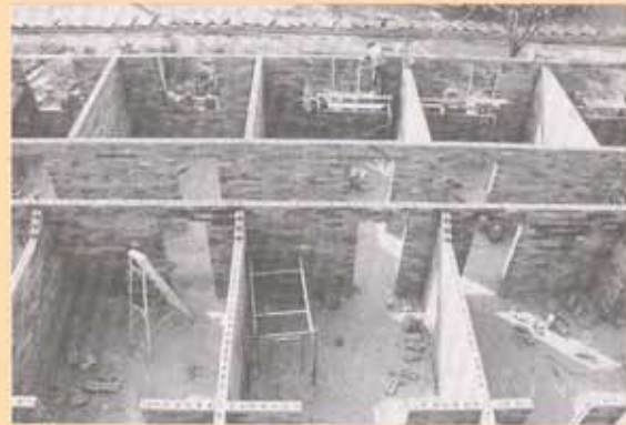
Above: Construction of the Aquaculture building using prefabricated building components developed and produced by the Habitech Center. Some of the prefabricated components are similar to those used in the Habitech demonstration house (right).
