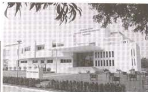
The Advance Agro Pulp and Paper Technology Building.
