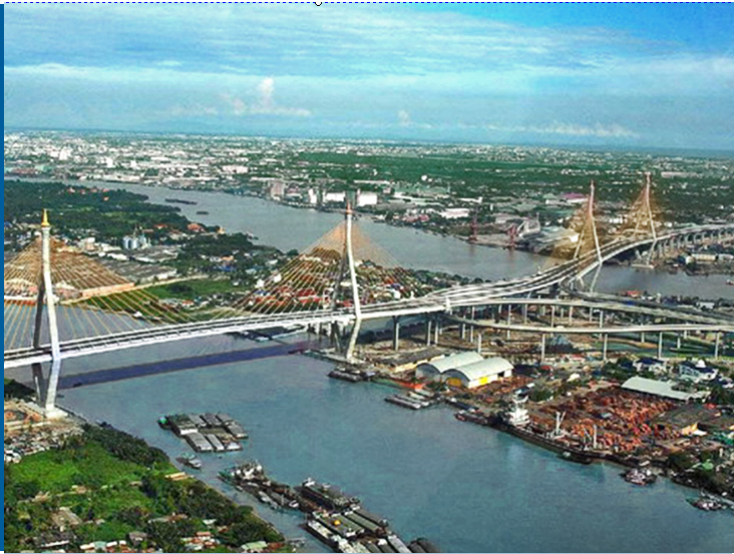
Industrial Ring Road Bridge, Bangkok
