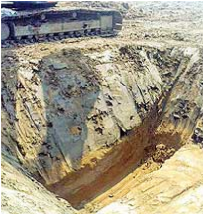
Excavation to test the connectivity of the trapped water.
