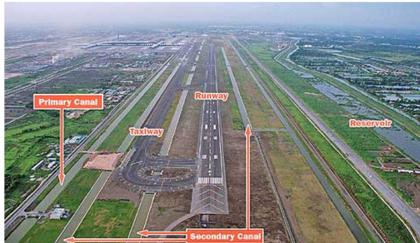
Overview of east runway, taxiways and the drainage system.
