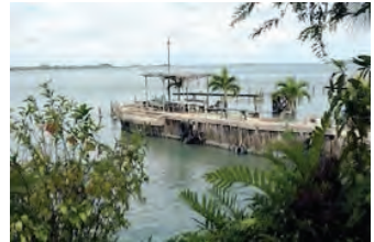
Evidence of coastal erosion in Paknamlaemsing District.
